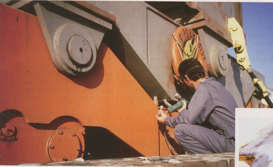
Inspector Richard Seals introduces non-destructive testing techniques and explains where to find fatigue cracks
