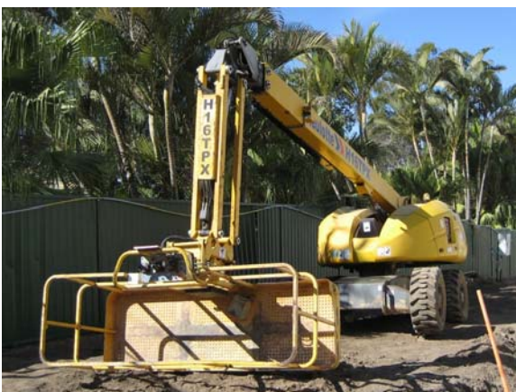
Photograph 1 – General view of EWP with platform hanging vertically
