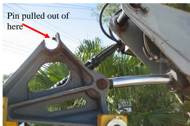
Photograph 2 – Close up of failed linkage
