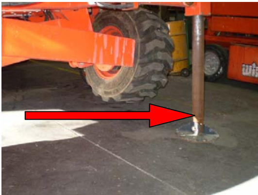
Use stabilisers to lift machine.
